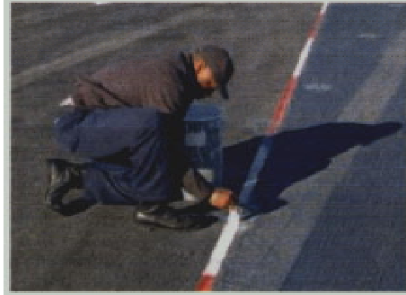
Figure 634-3-13. COLOR TOPPING APPLICATION
